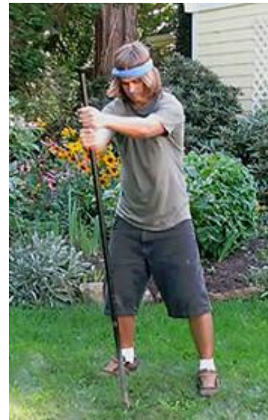
Preparing a Post Hole with a Digging Bar
